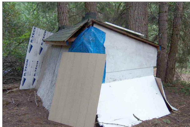
Figure 2. Exterior of Ventilated Thermal Shelter under a heavy tree canopy, with air-gap double-walls and protective shade panels.
