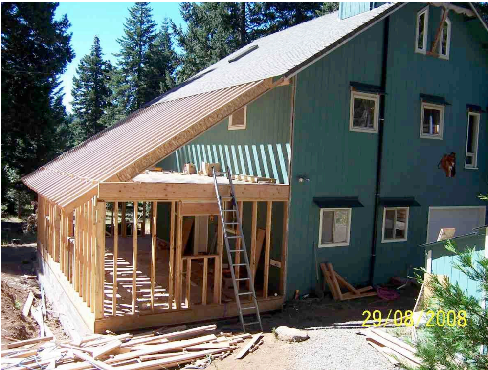
Photo: New construction at OBRL
