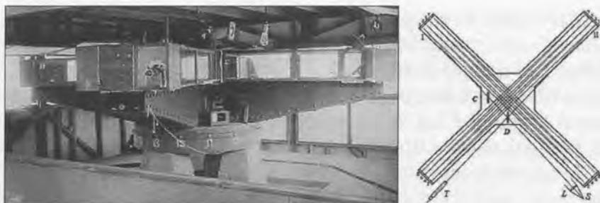
Figure 1. Miller's interferometer (left). Light paths of the Michelson-Morley and Miller Interferometers, as seen from above (right).
